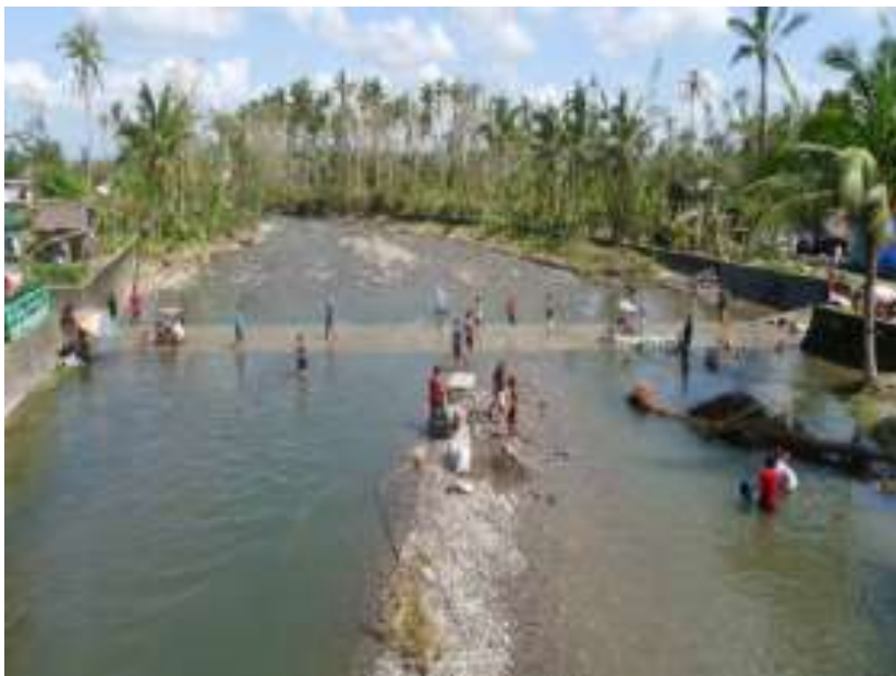
PONGSO RIVER WITH DISCHARGE OF 43-70 MLD
