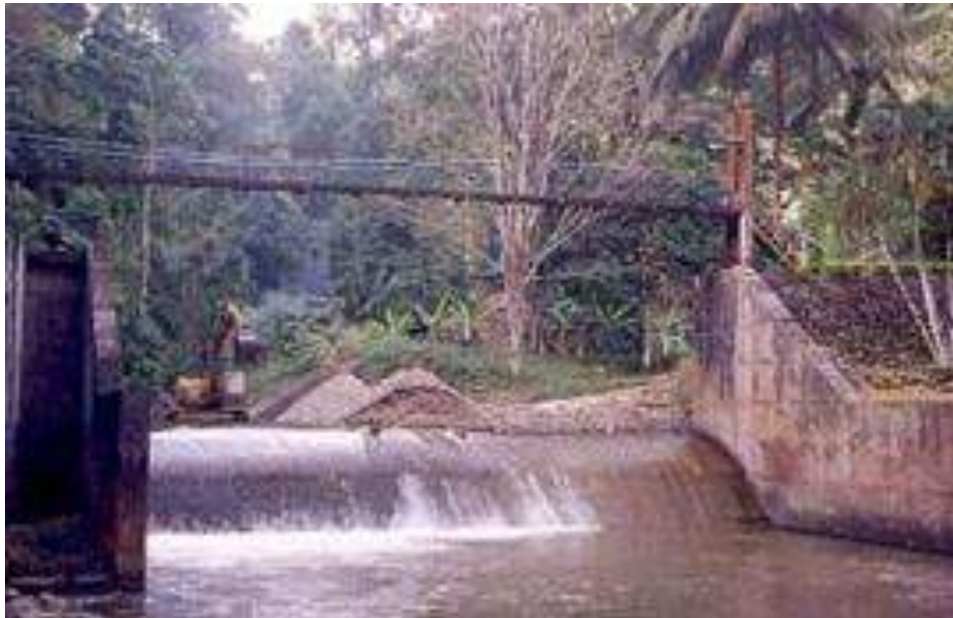
EXISTING SOURCE OF ZCWD IS A DIVERSION WEIR AND NO HOLDING CAPACITY, THUS, WATER IS WASTED DURING RAINY SEASON AND THE WEIR RUNS DRY DURING SUMMER EXACERBATED BY EL NIÑO.
