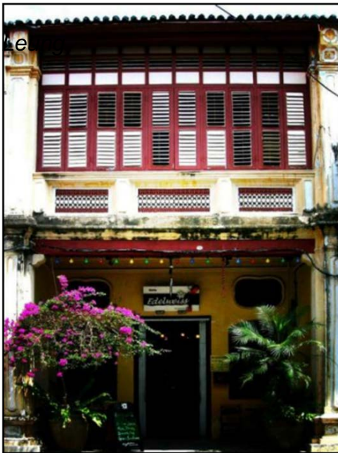
Heritage shophouse, Malaysia.
