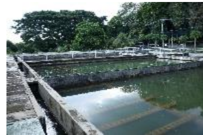
WATER TREATMENT PLANT AT PASONANCA
