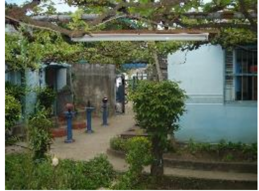
SEWERAGE PUMPING STATION
