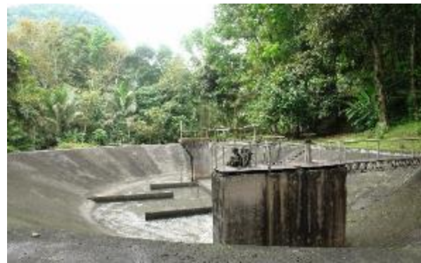
OLD RESERVOIR (LEFT) SAND AND GRIT REMOVAL BASIN (RIGHT)
