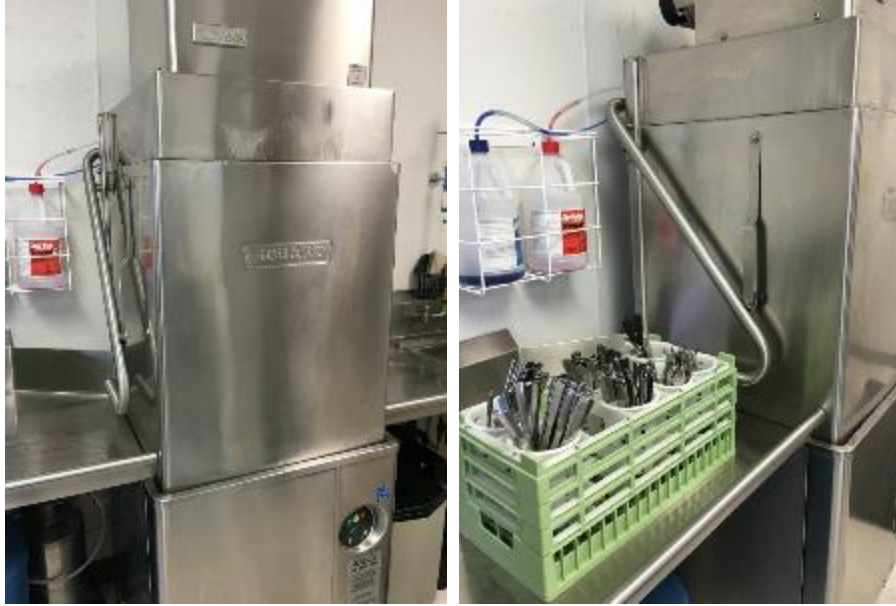
STATIONARY HOOD TYPE DISHWASHER
